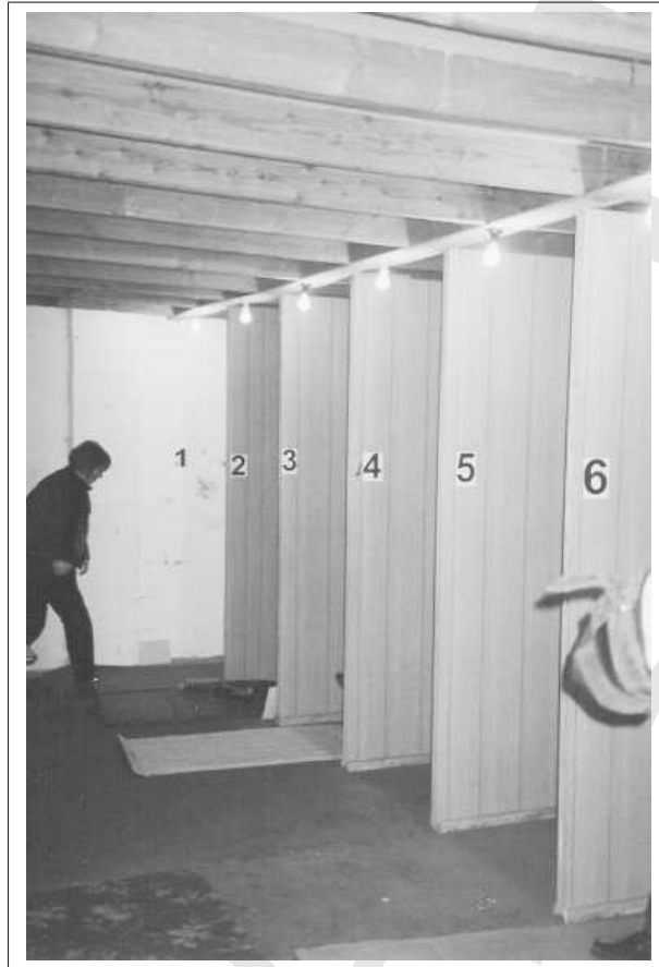
Figure 41: Rathdrum Rifle and Pistol Club. View of Firing Line. Note the individual baffles fitted to each firing point.
